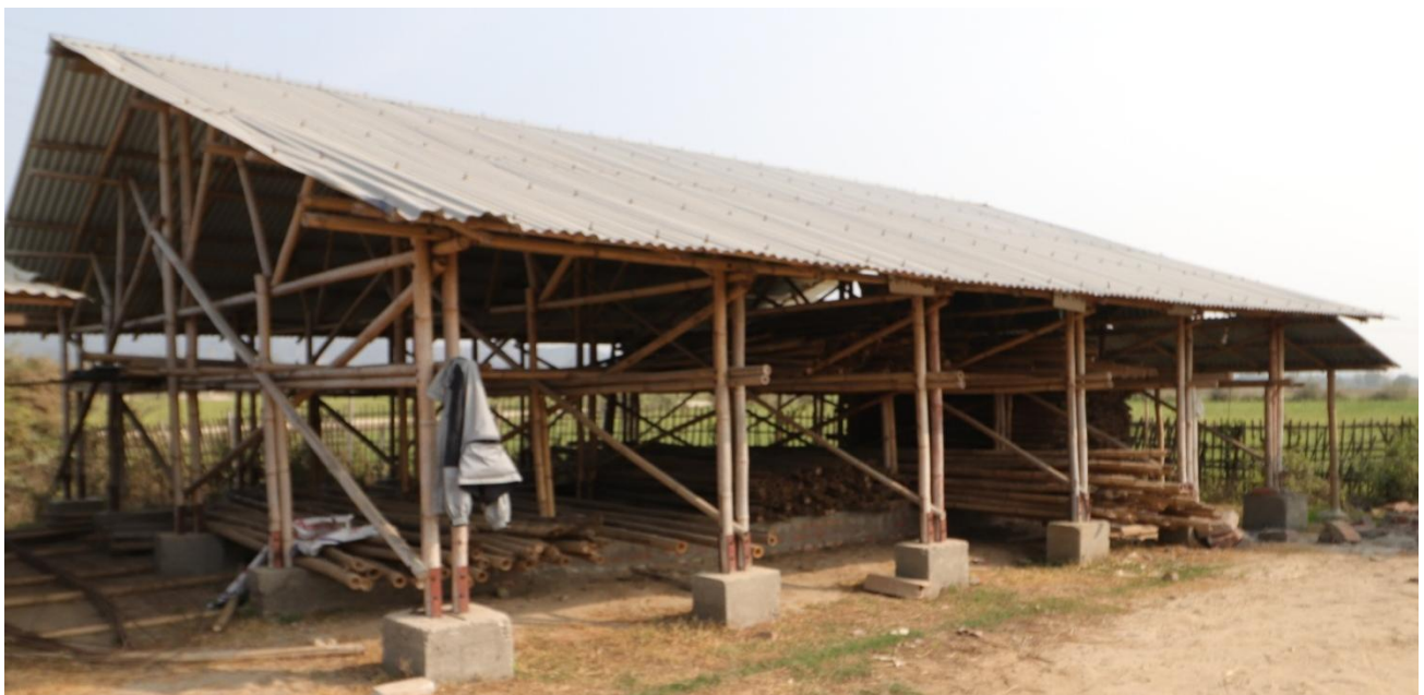
Figure 1: Example of Bamboo Braced Frame System
