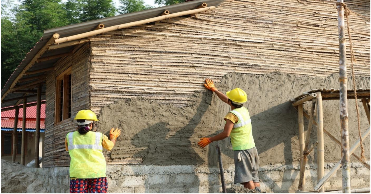
Figure 2: Example of Light Composite Bamboo Shear Wall (CBSW) System
