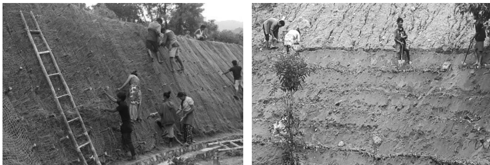
Figure 6 - Bio-engineering work in Sankhu-Palubari-Nagarkot Road
