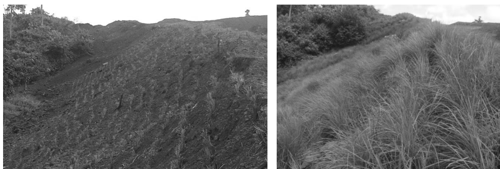
Figure 3. Grass plantation in mine haul road in Tokadeh, Liberia (before and after 3 months)
