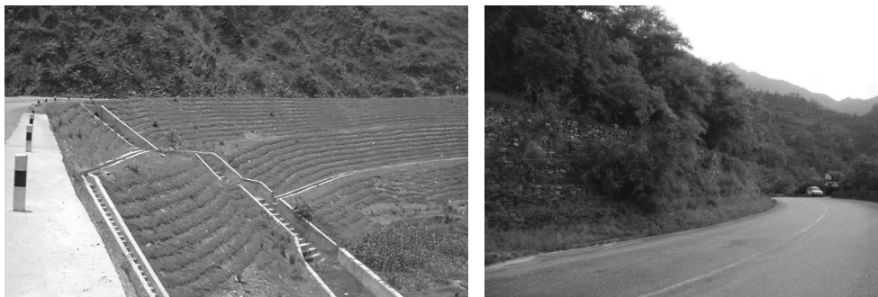
Figure 4. Combination of civil and bio-engineering techniques in Nepal road
