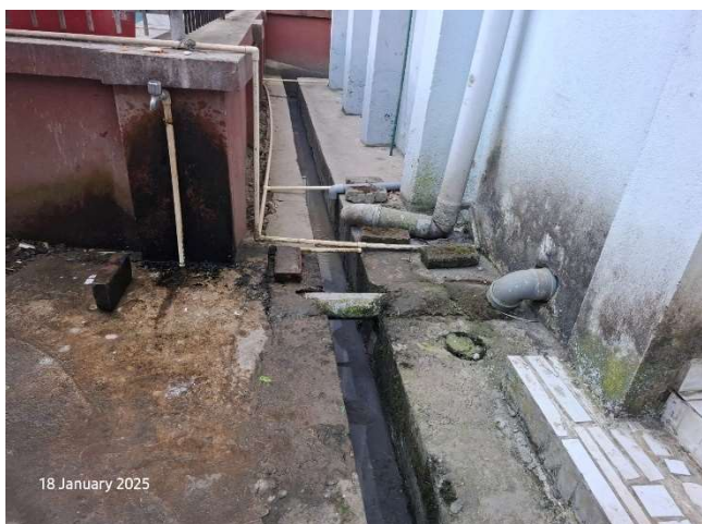
External drains uncovered.
