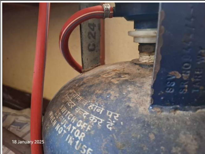
Expired LPG cylinder being used.
