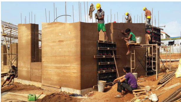
(a) Rammed Earth Wall
