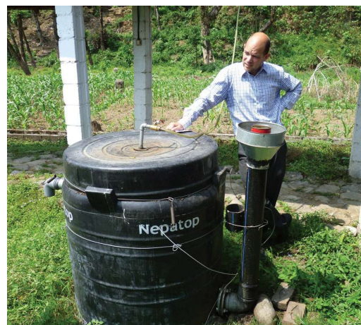
(b) Plastic stacked barrel biogas plant.
