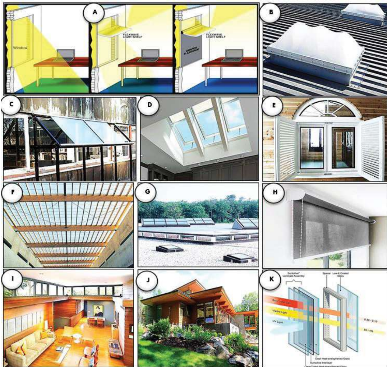
Fig. 3. Some of traditional daylighting applications/methods; (A) Window and light shelf, (B) Prismatic glazing, (C) Holographic films, (D) Skylight, (E) Metal louver, (F) Translucent roof, (G) Roof monitor, (H) Roller blind, (I) Clerestory window, (J) overhangs, and (K) Assembling glazing [50-53].
