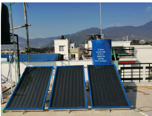
Figure 69: Passive Solar Water Heating System
